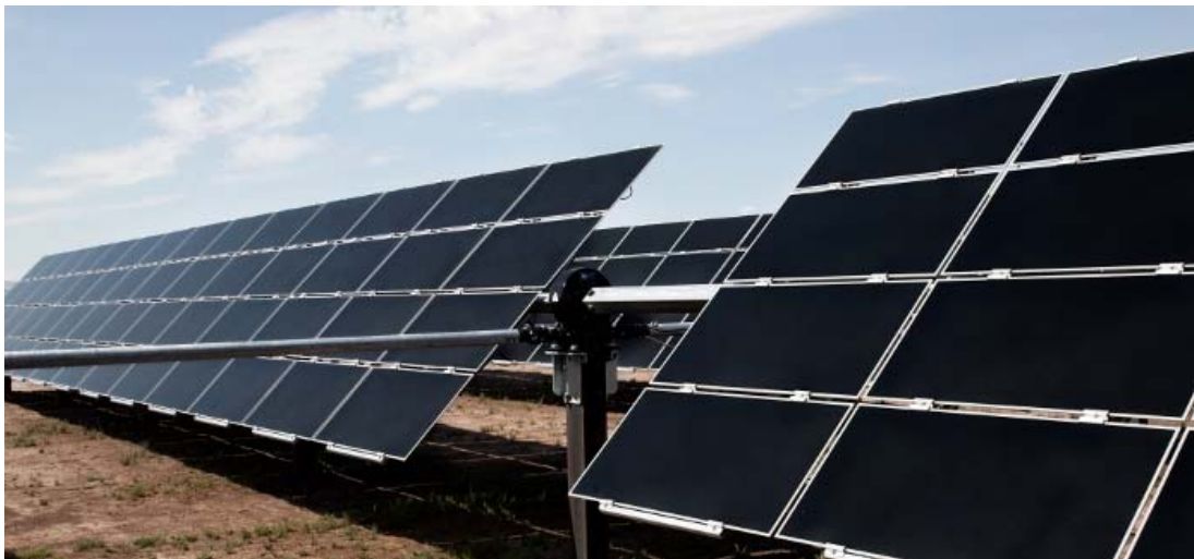
Plate 2. Example of a typical frameless solar array mounted on a single axis tracking system 8
